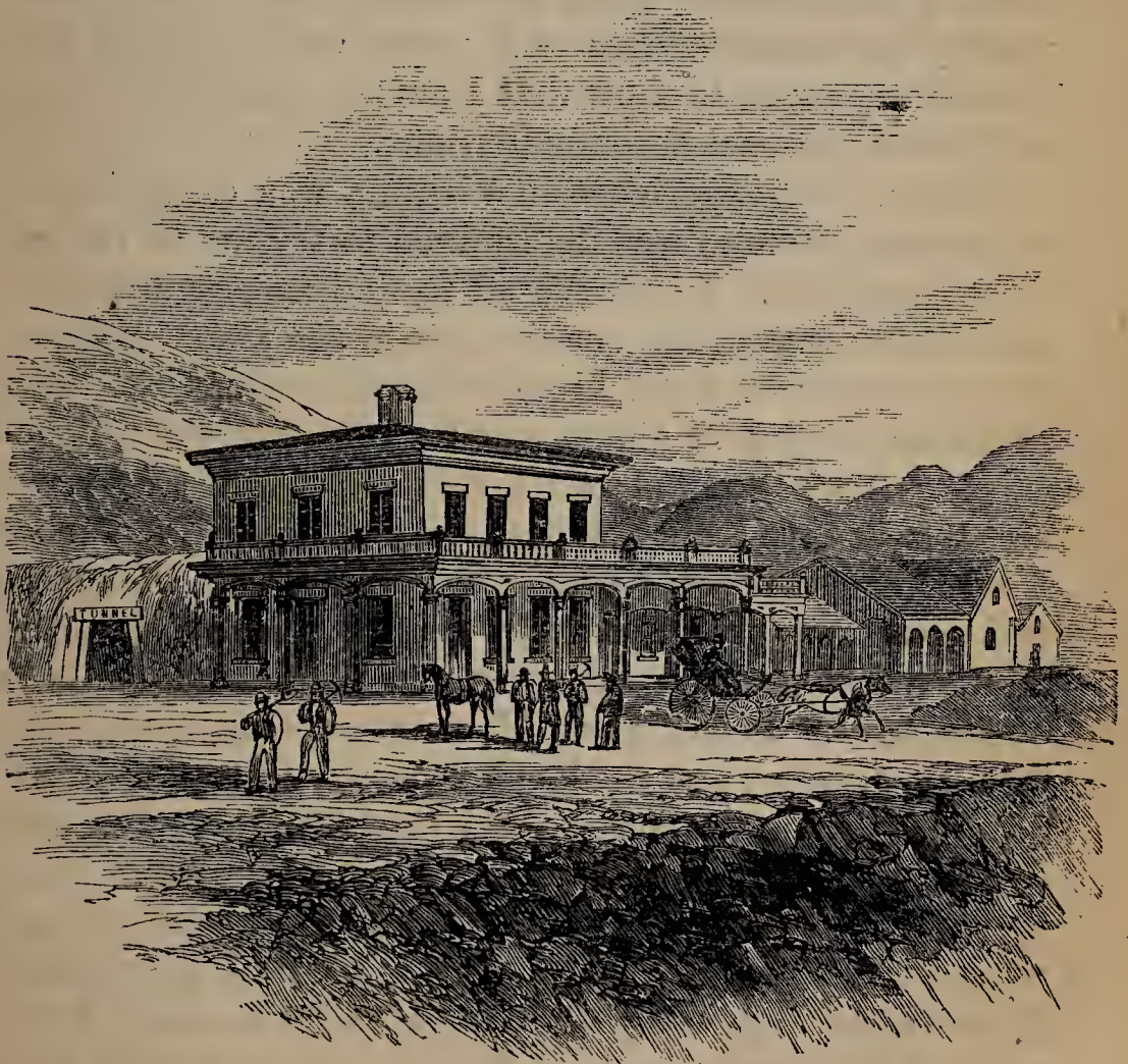
OFFICE AND DWELLING OF THE GOULD AND CURRY COMPANY.
